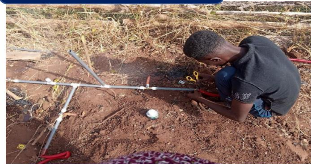
Plumbing works at site
